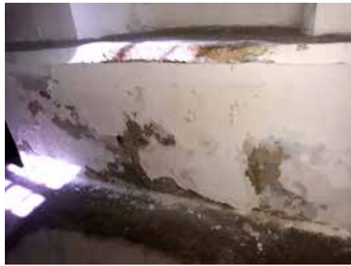
Fig.2 – The state of the altar apse during the 2011 year with increased moisture
