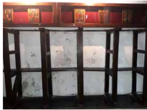
Fig.2 – The state of the altar apse during the 2011 year with increased moisture
